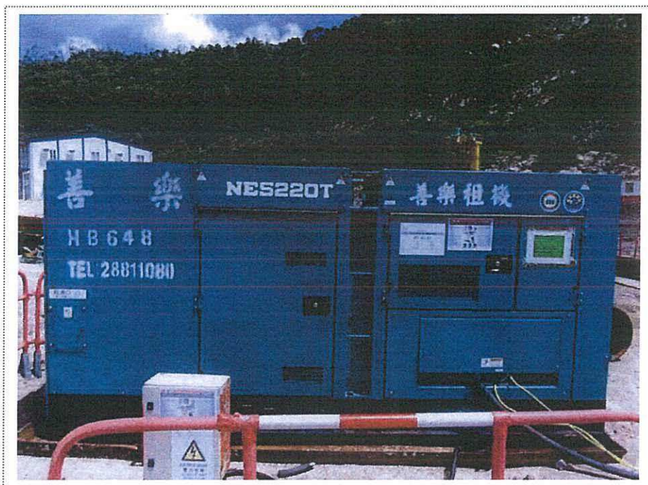
Generator, with Quality Powered Mechanical Equipment Label showing a Sound Power Level \leq 94 dB(A)
